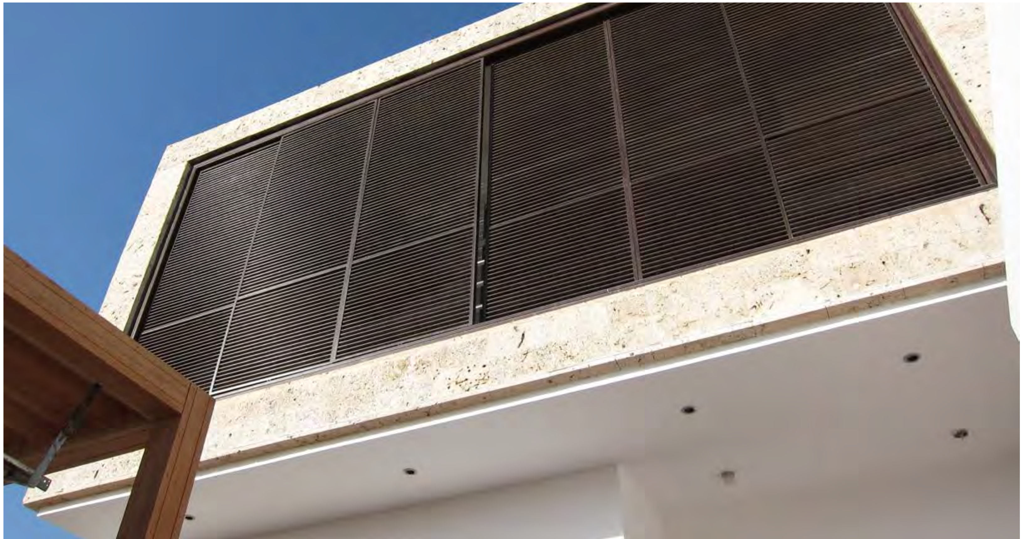
Al-Wesal Semi Detached Units Jeddah
