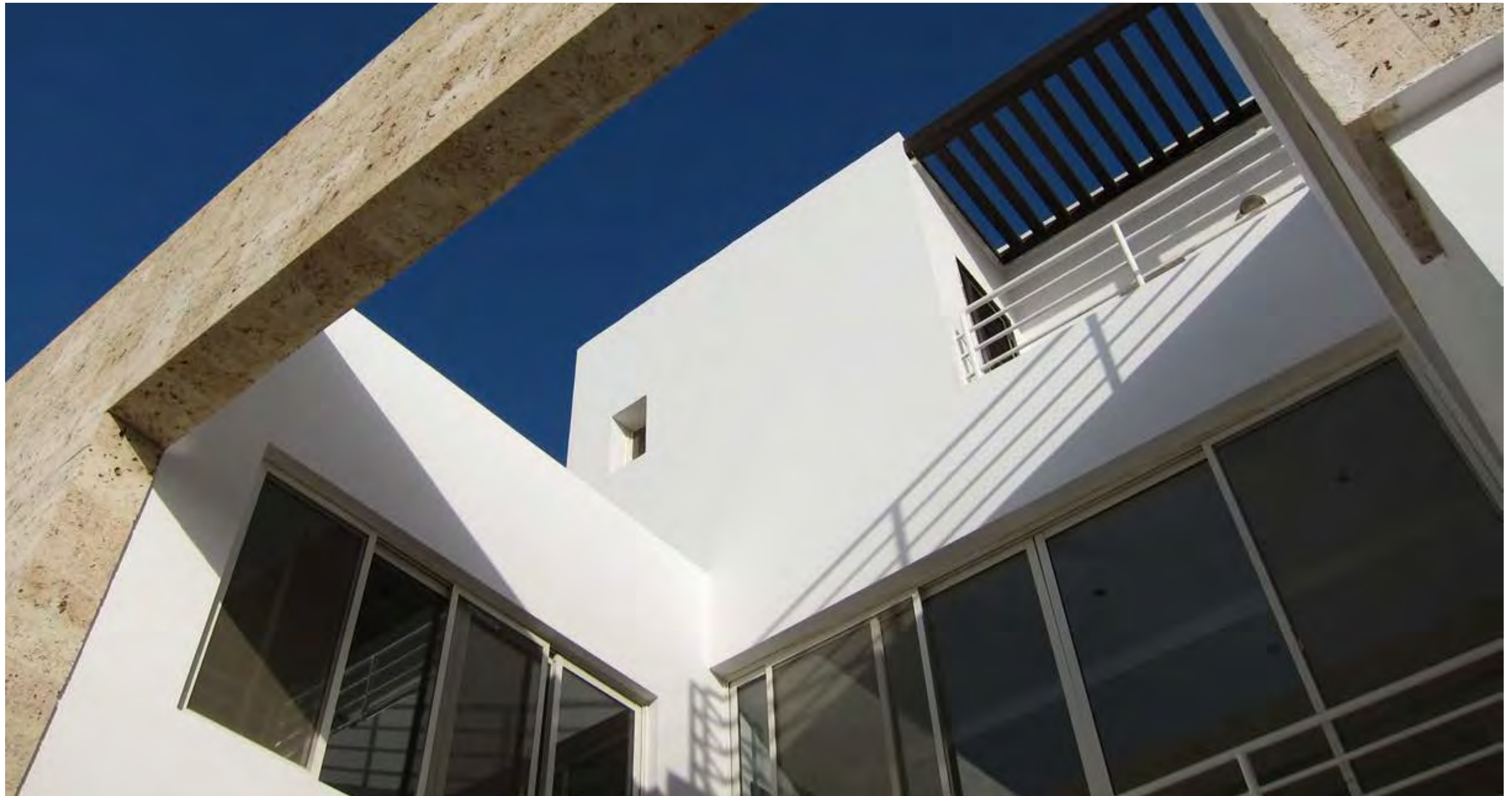
Al-Wesal Semi Detached Units Jeddah
