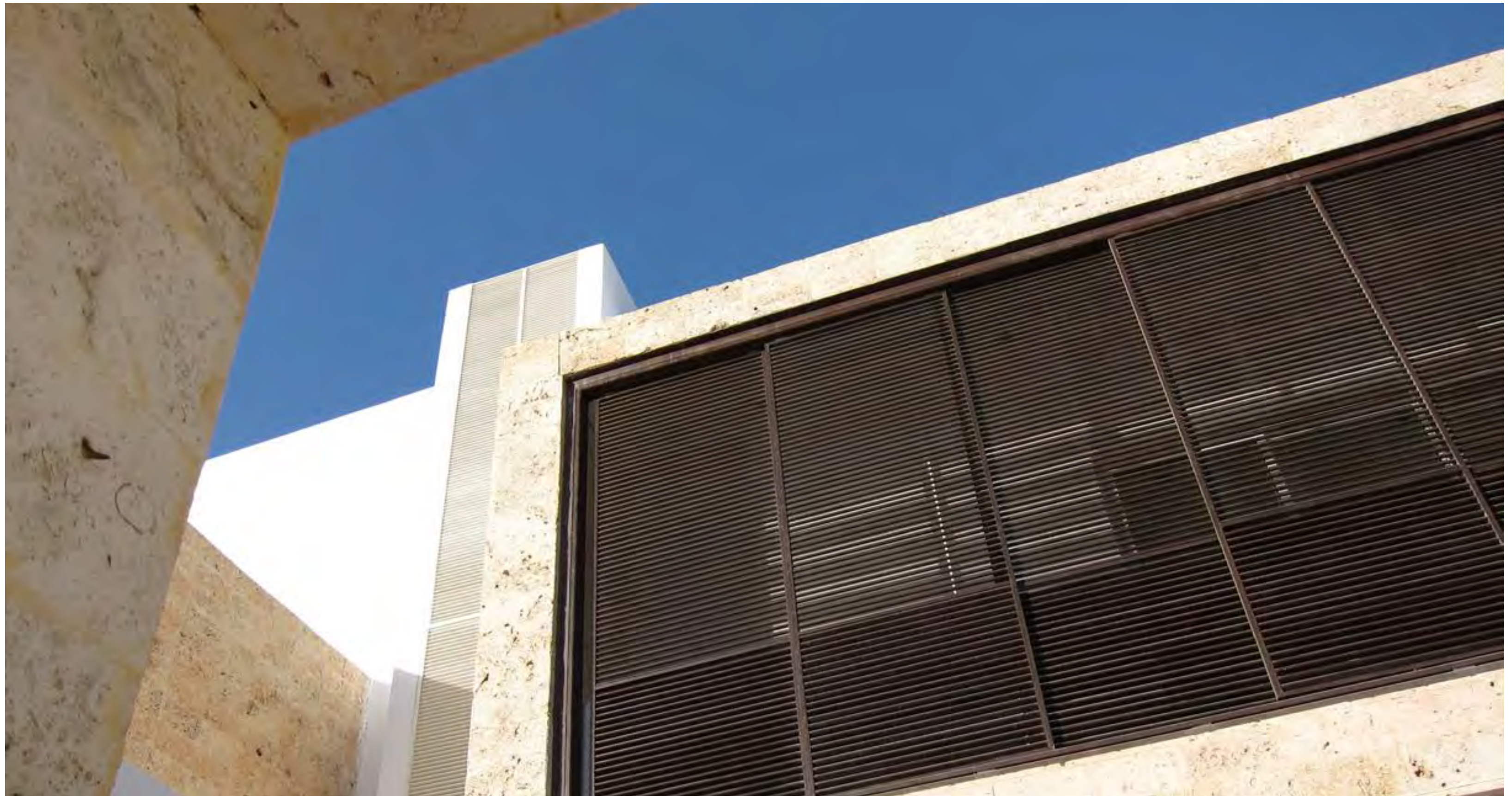
Al-Wesal Semi Detached Units Jeddah
