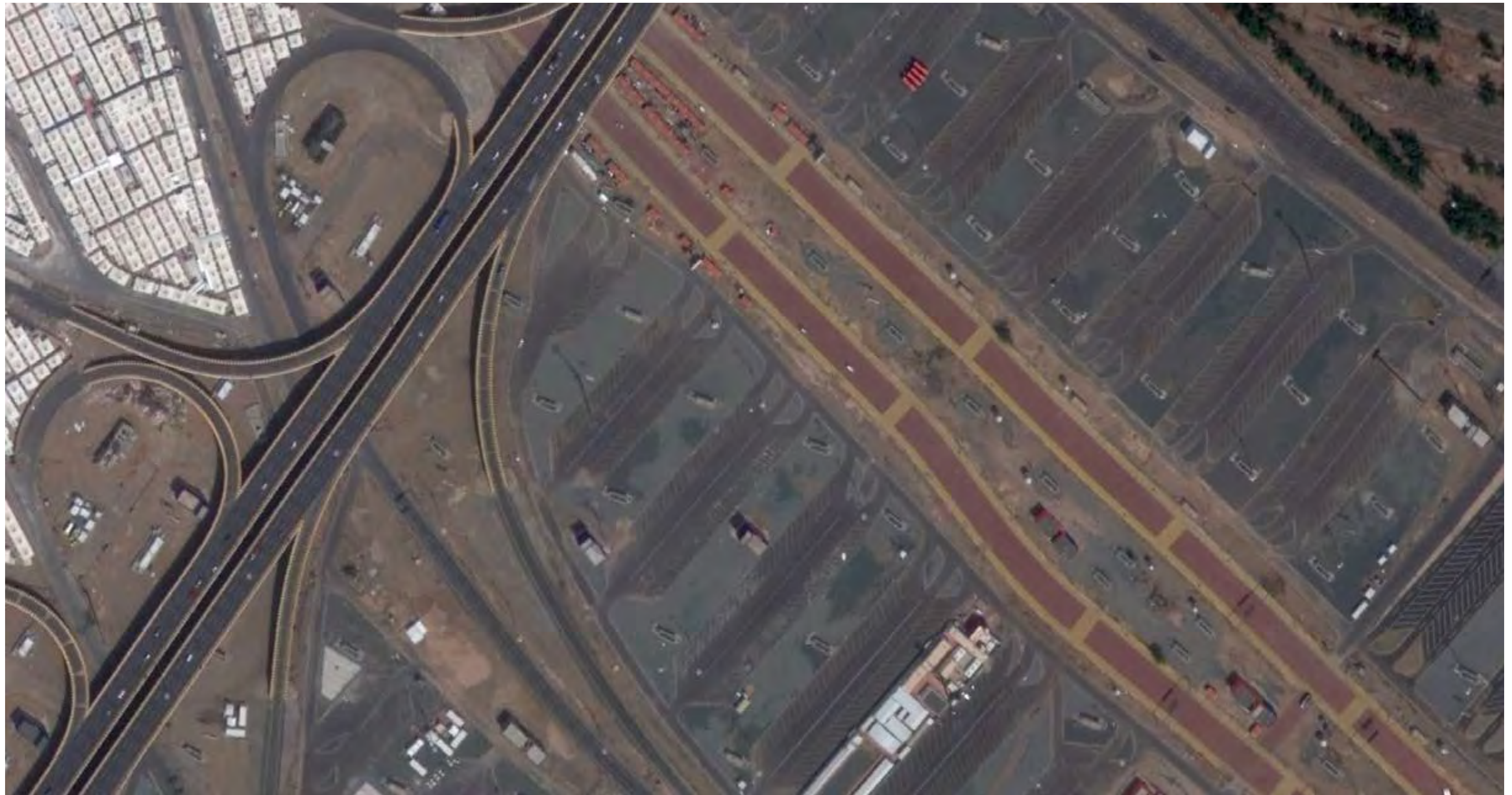
Muzdalifah Walkway Shading Makkah
