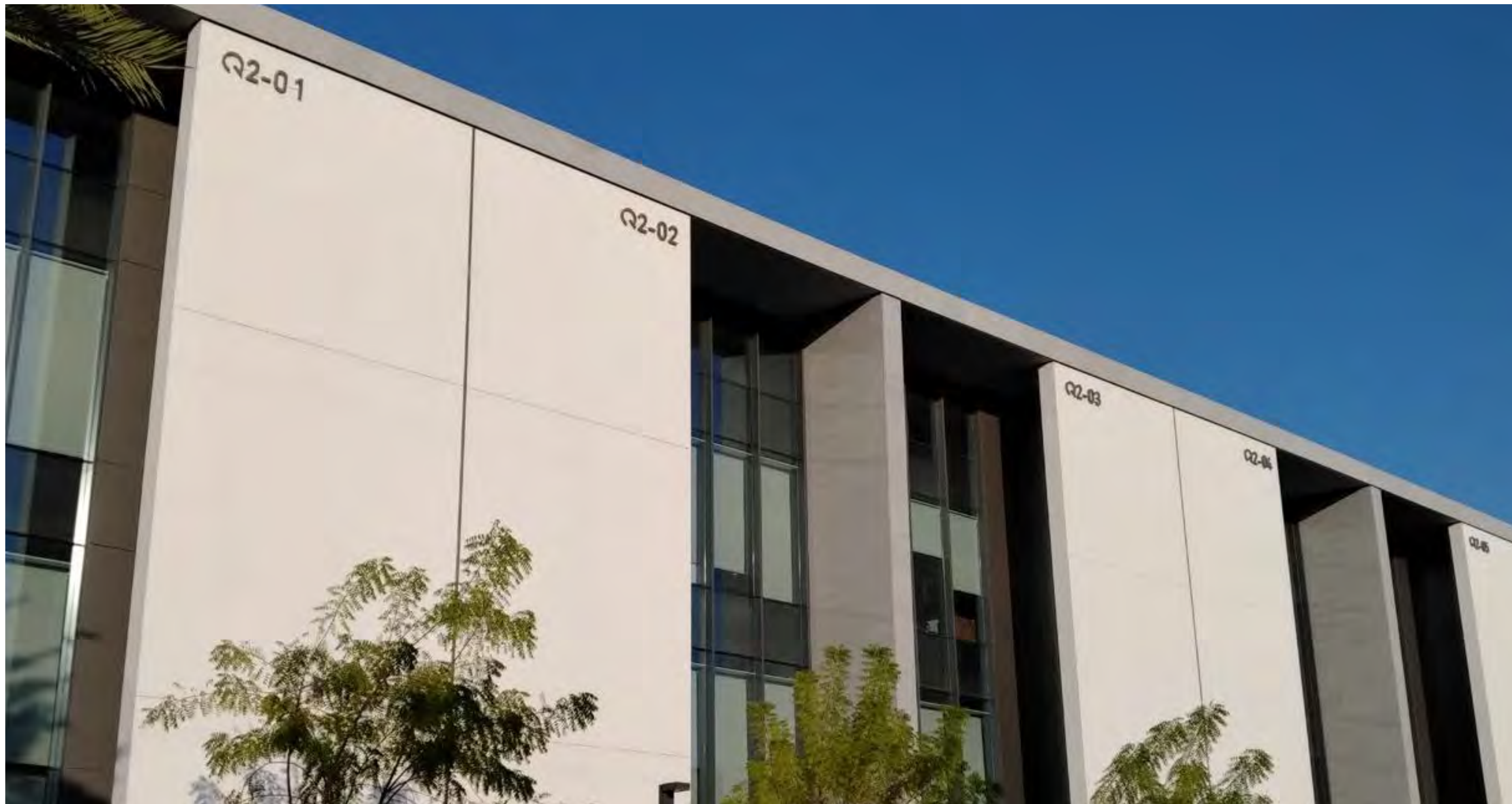
BQ – Office Park Dammam
