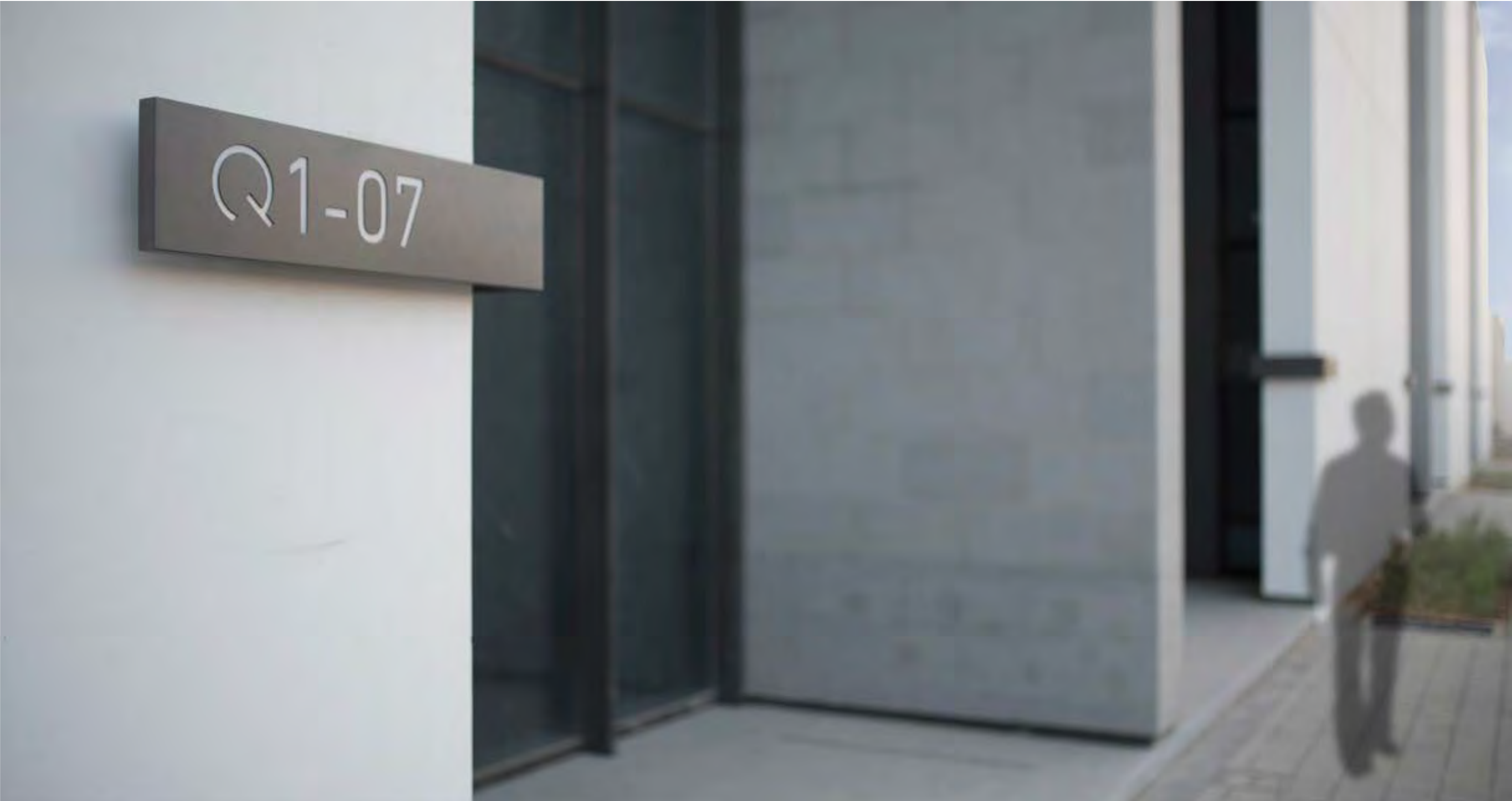
BQ – Office Park Dammam
