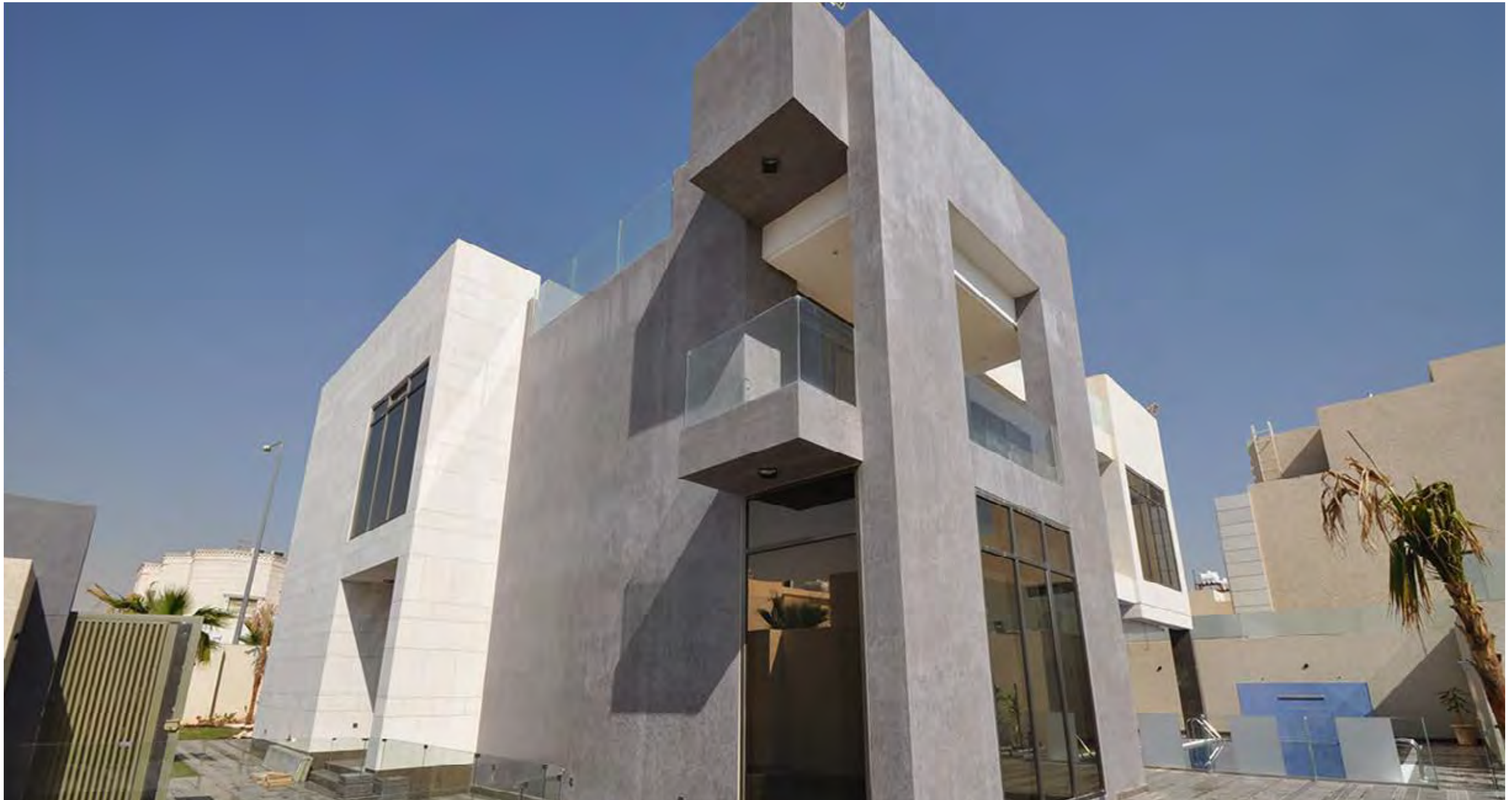
Al-Mane'e Residence Complex Riyadh
