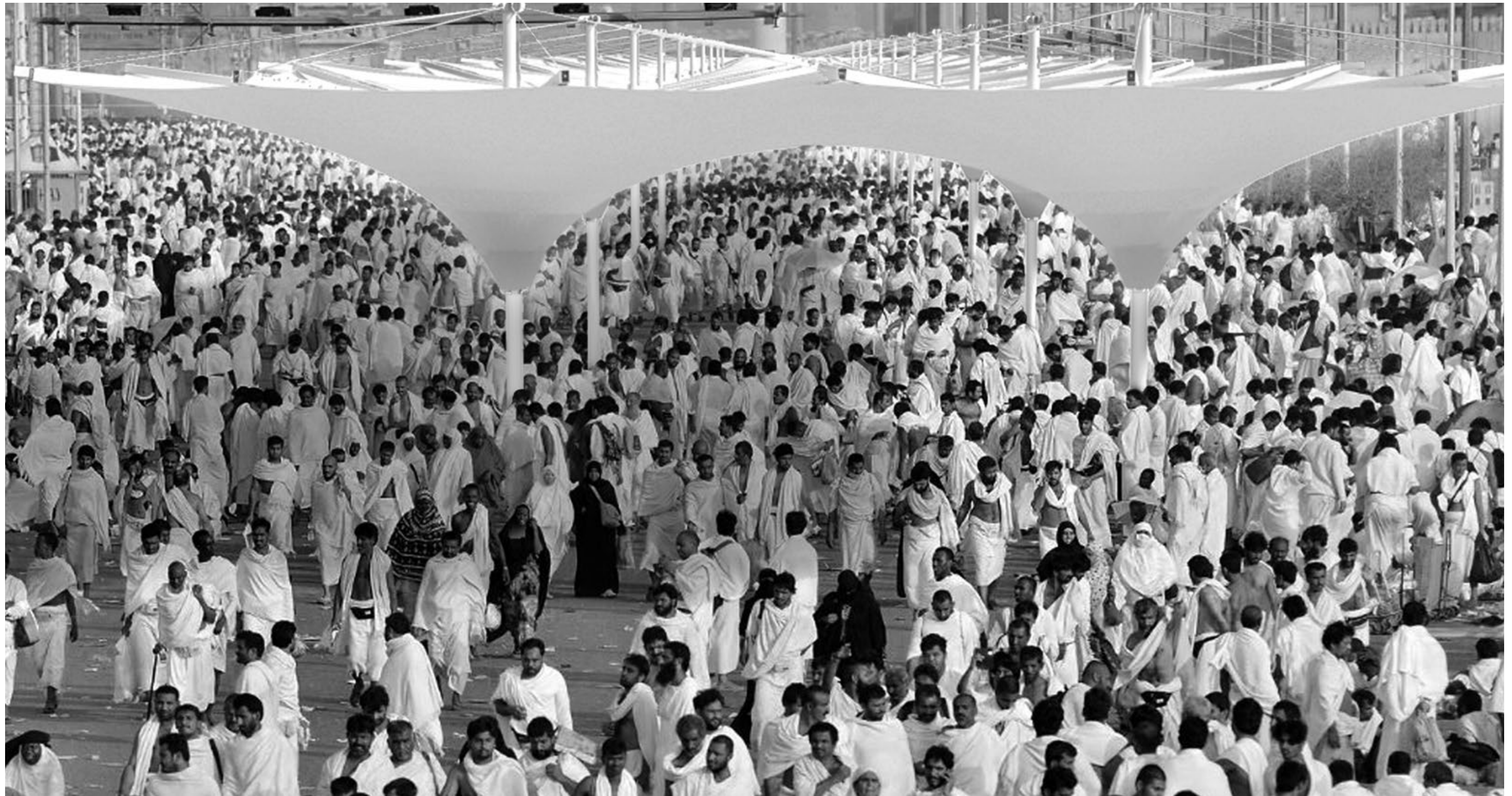
Muzdalifah Walkway Shading Makkah
