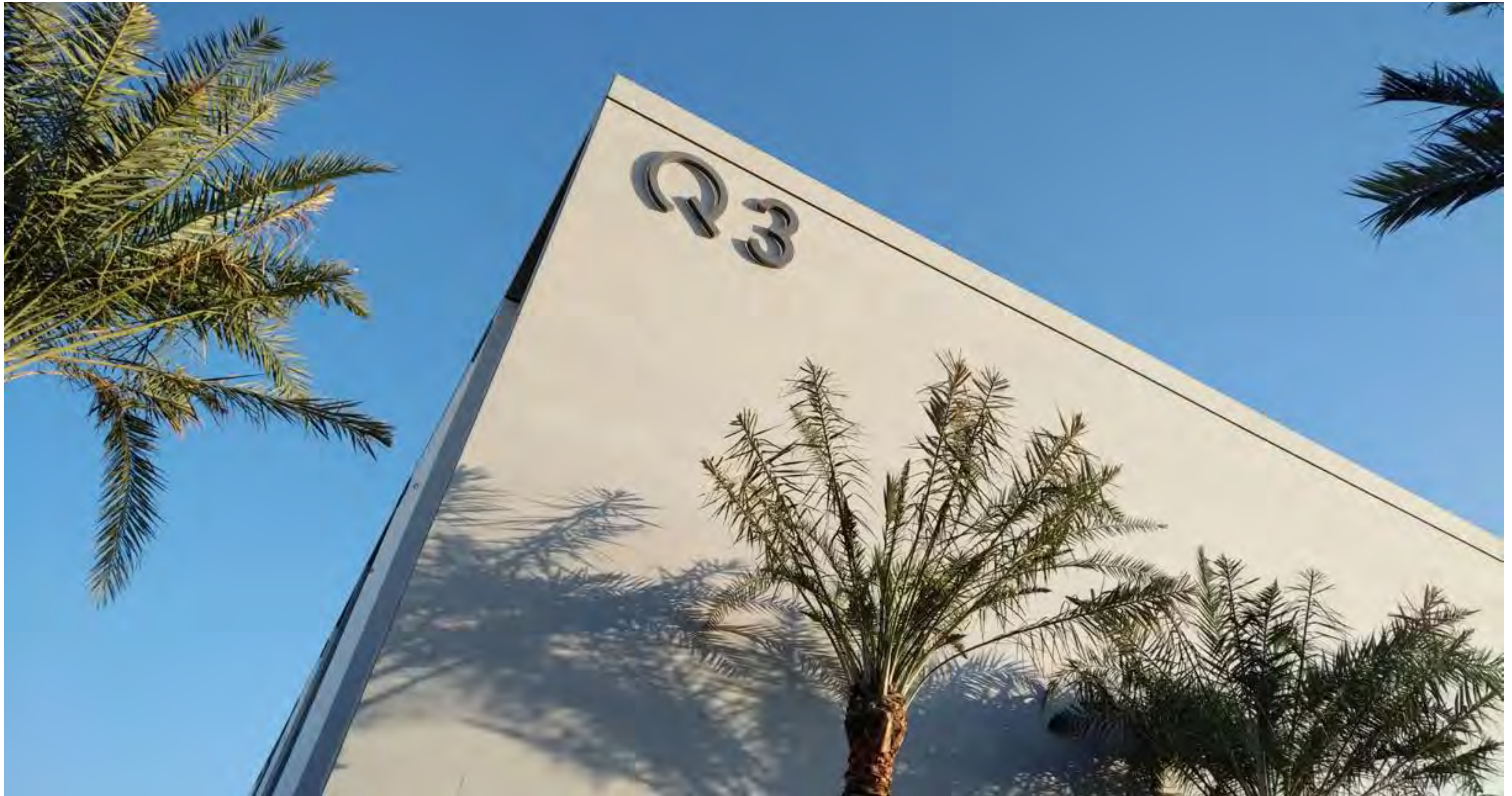
BQ – Office Park Dammam
