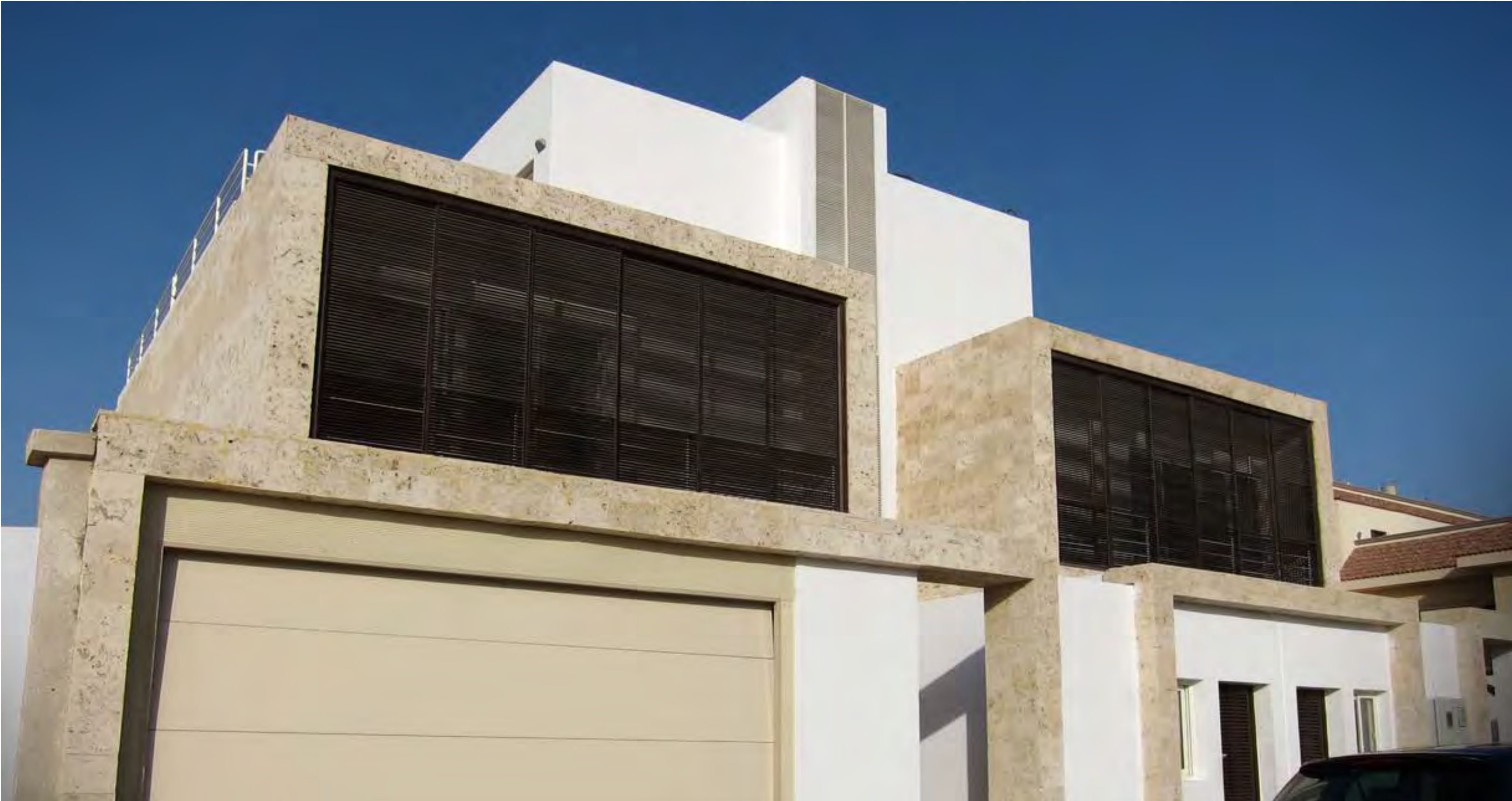
Al-Wesal Semi Detached Units Jeddah
