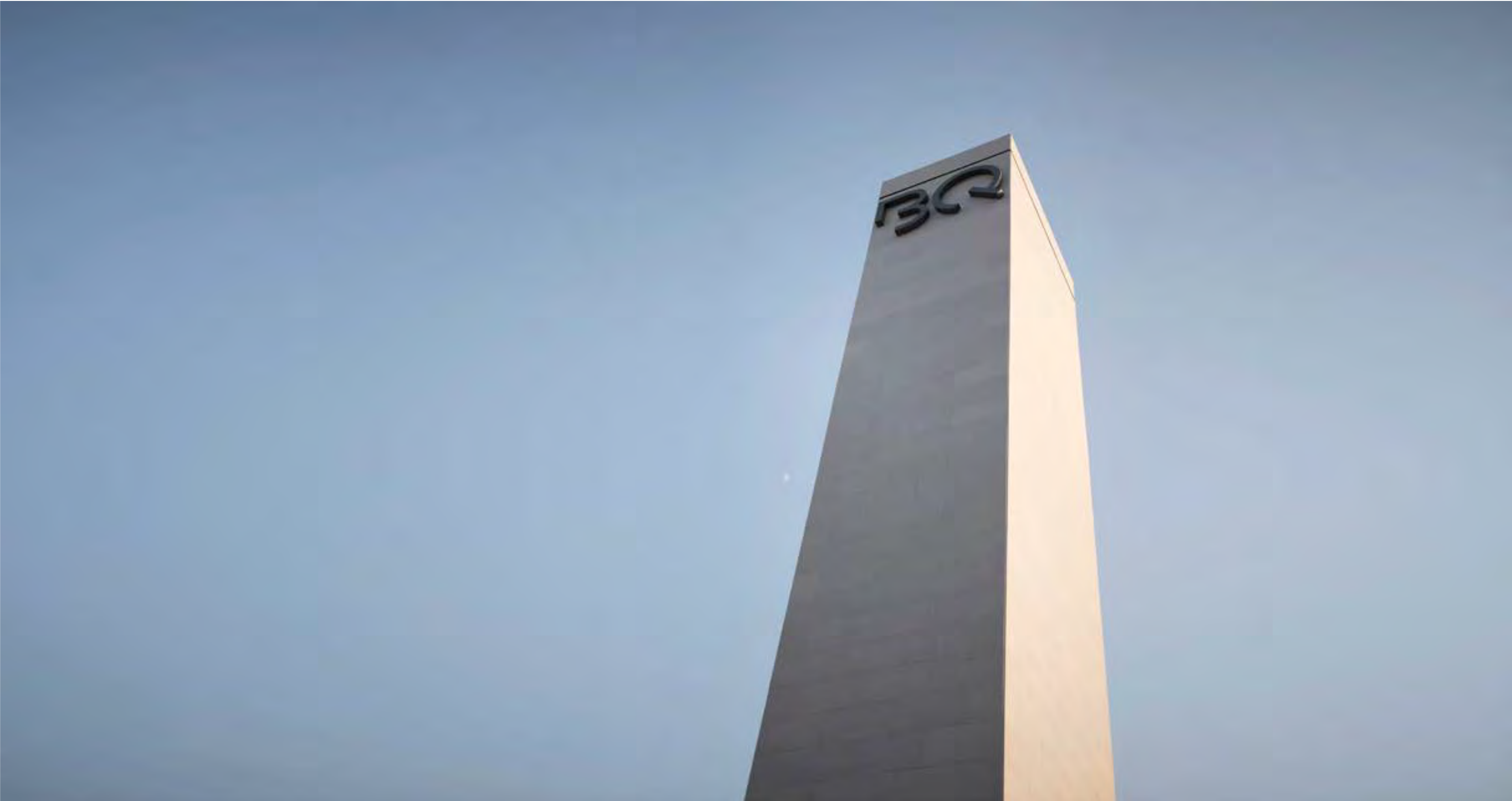
BQ – Office Park Dammam
